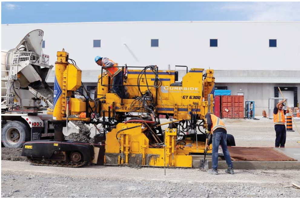
Curbside Construction purchased their first Commander III (GT-6300) in 1987 and the company still uses it today on different projects. Their inventory of GOMACO equipment has grown over the years to include not only GT-6300s, but multiple GT-3600 curb and gutter machines and a GT-3200 sidewalk paver.
