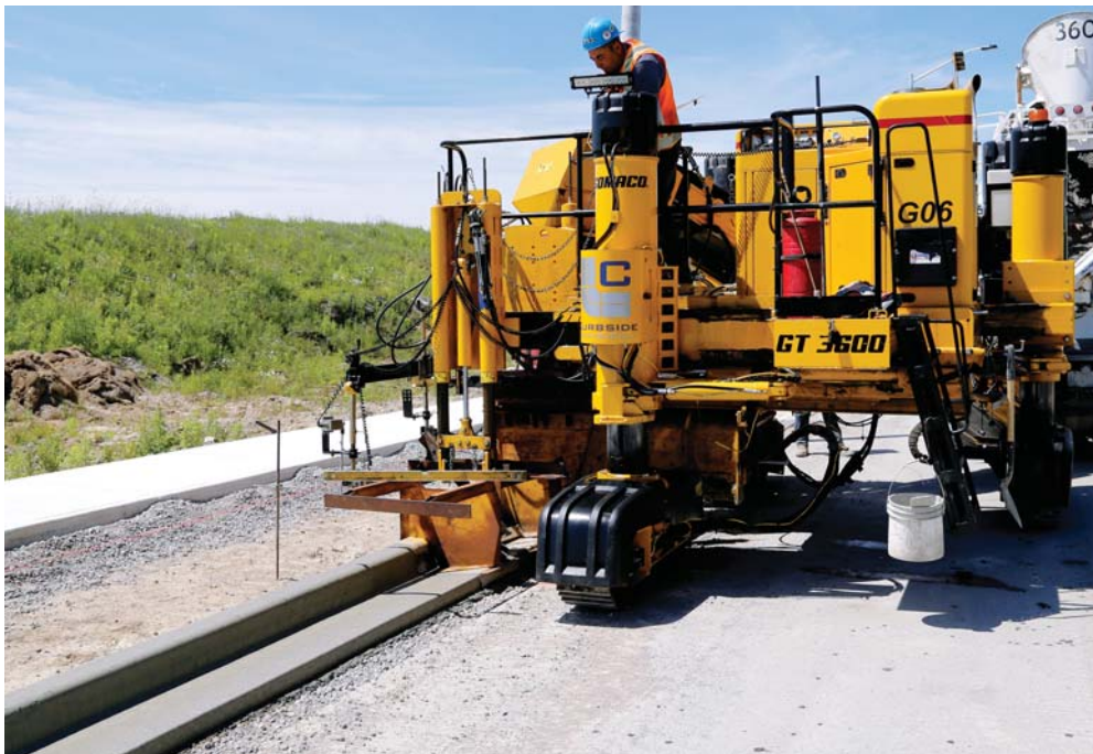
Curbside has three curb and gutter crews at work on a daily basis slipforming a variety of profiles. Here, a GT-3600 slipforms the curb and gutter portion of two-stage curb on a new road for a subdivision.
